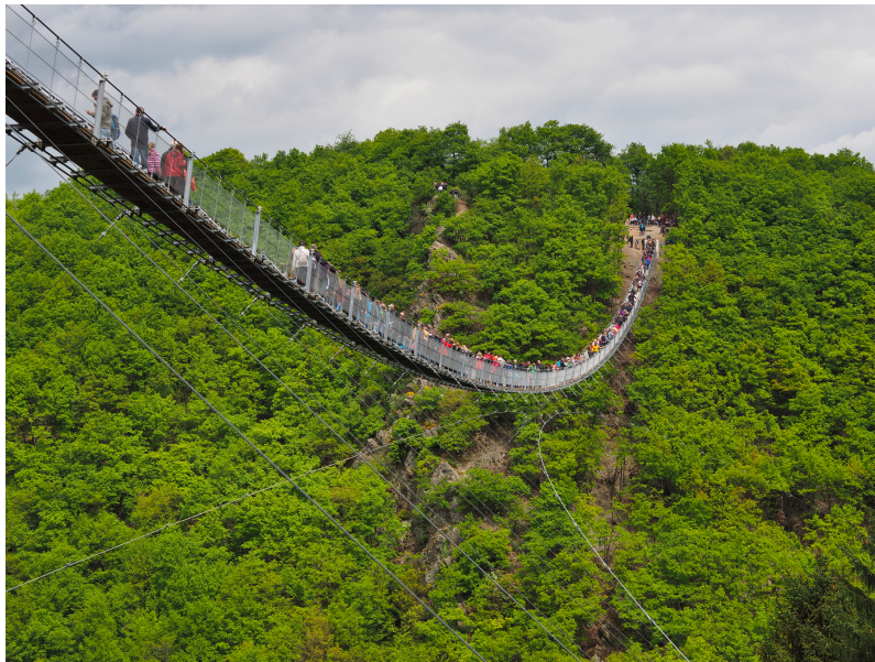
Figure 5: The Geierlay suspension bridge in Western Germany ("Geierlay").
